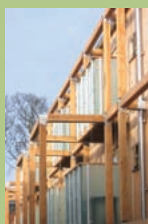
Showing structural framing for 'green planting'
