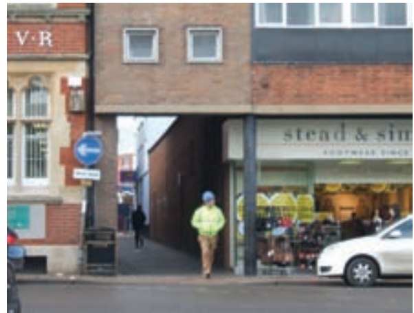
1. One of the unsatisfactory passageways linking The Arc development to the existing shopping centre of Bury St. Edmunds
