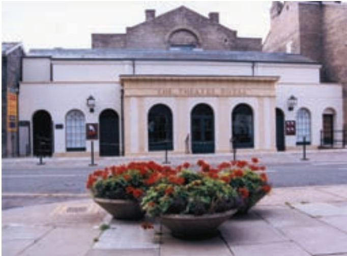
Front elevation before 2005
