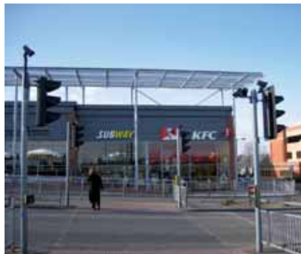
5. The corner unit steps back to provide a little extra visibility at the exit from the car park – but the fence obscures car drivers’ sight lines. Also a canopy runs over the whole frontage – is this trying to tie the fragmented façade together? It certainly will not keep out the rain.
