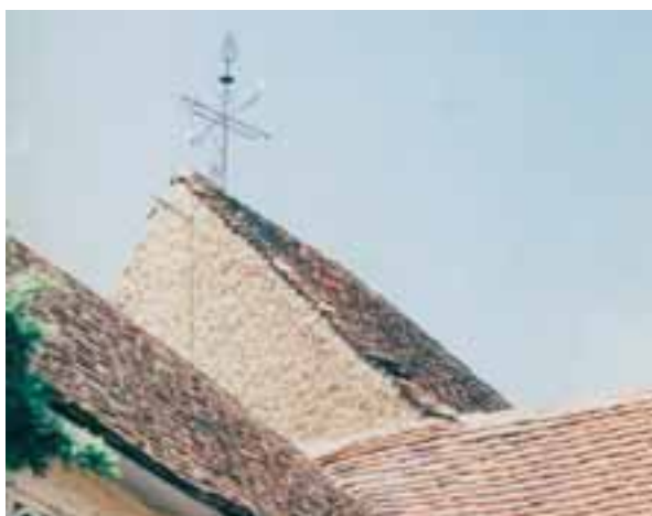
'Pebbledash' facing on the gable end of The Great House Restaurant, which adjoins Little Hall.
