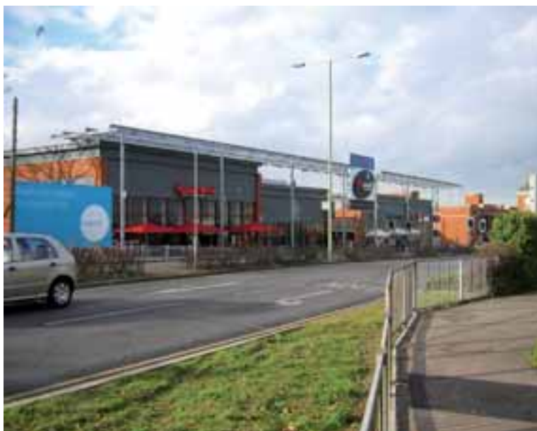
The cinema's siting at the road junction – 'a bright, vibrant and active frontage'?
