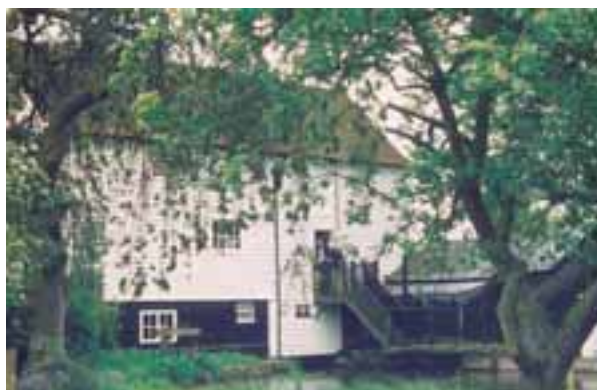
The newly lime washed exterior of Pakenham Water Mill
