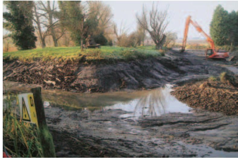
During work of dredging – December 2005.
