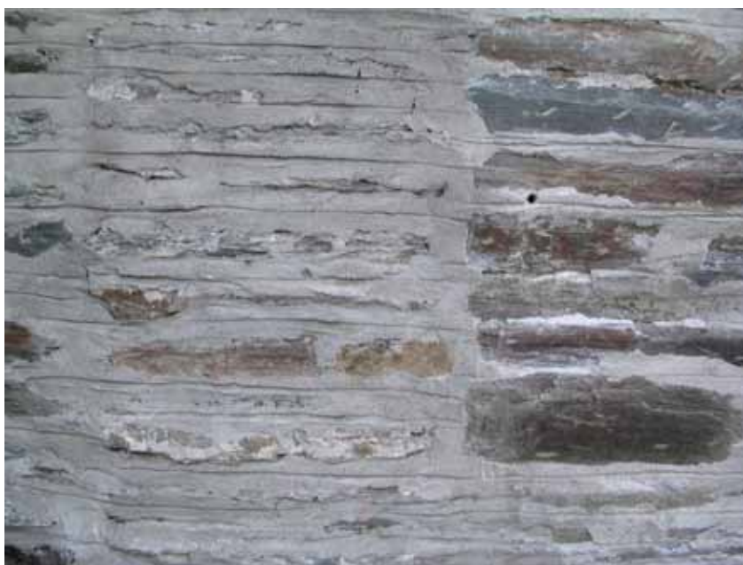
Note the difference on this stonework when the loose mortar is removed (on the right-hand side) which indicates that re-pointing was unnecessary.
