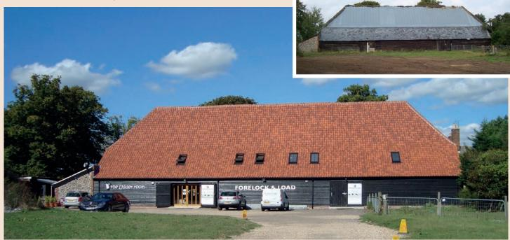
A large semi-aisled barn dating from the early C19th, this was added to the At-Risk Register in 2000 following deterioration of the thatched roof. Consent was granted for conversion to office use, but this was not implemented. Following a new consent, the barn has been converted to a retail outlet for equine accessories, with the village
